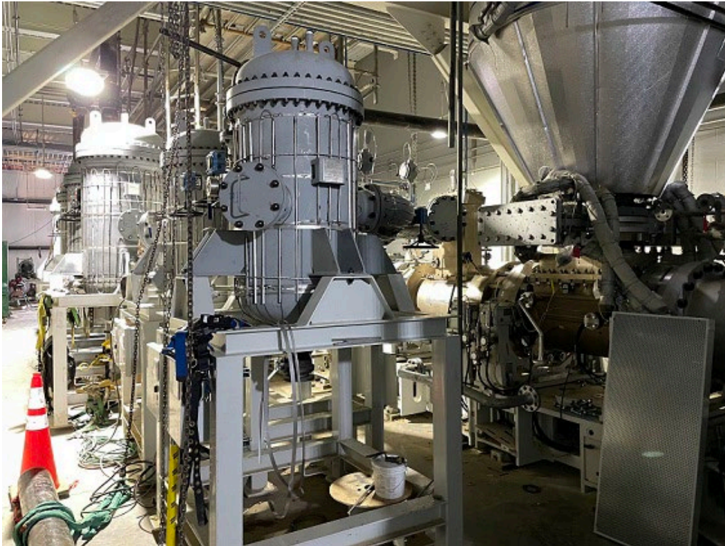
Figure 4: Installation of Extruder Dust Collection Piping in Building 610
