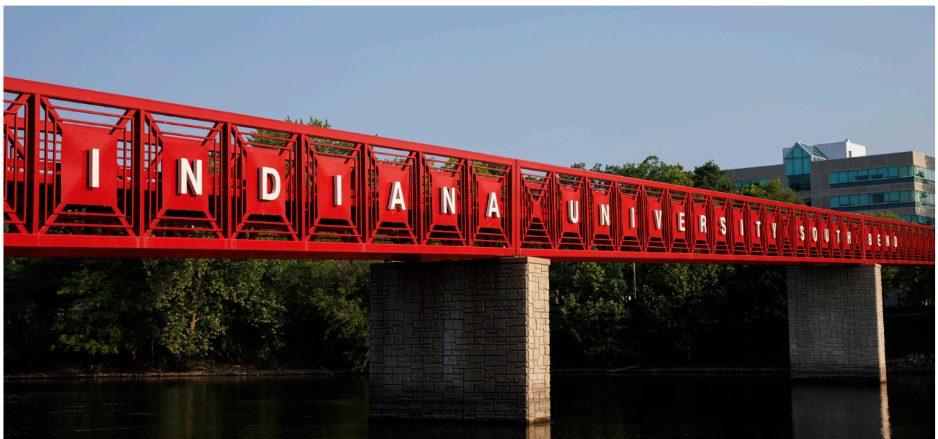
Pedestrian bridge across the St. Joseph River IU South Bend Campus
