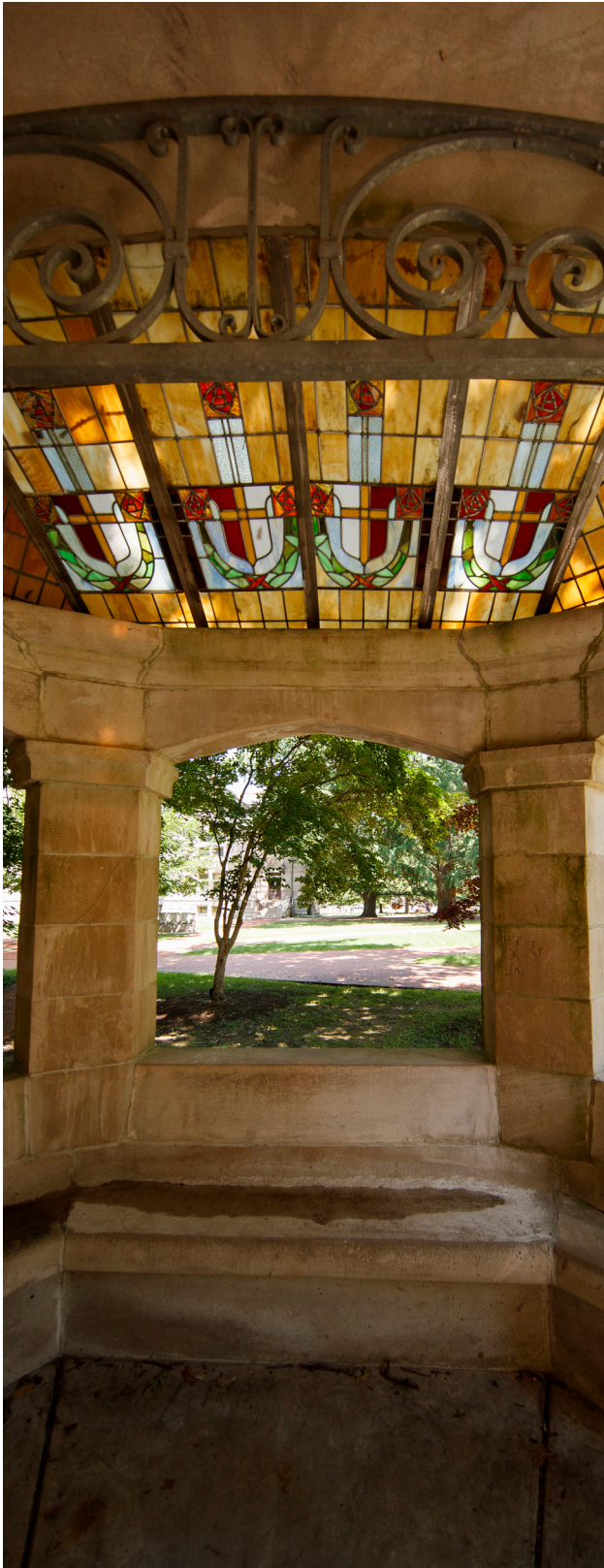
View from inside the Rose Well House IU Bloomington Campus
