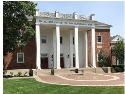
Halbritter Center for the Performing Arts
