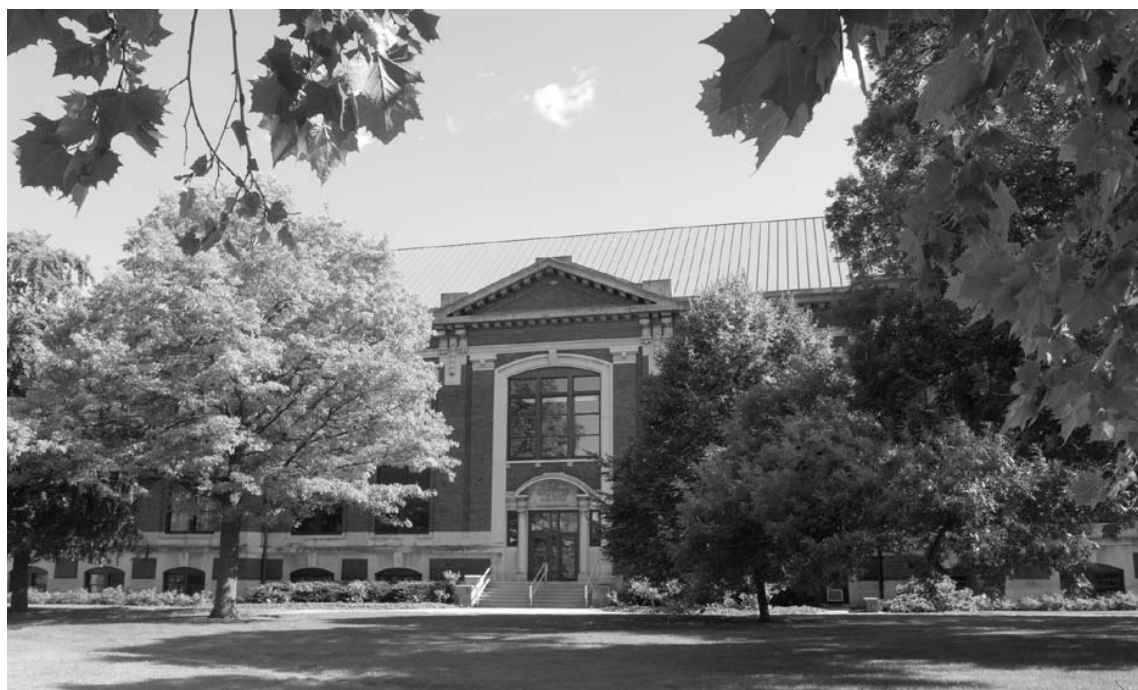
Agricultural Administration Building
