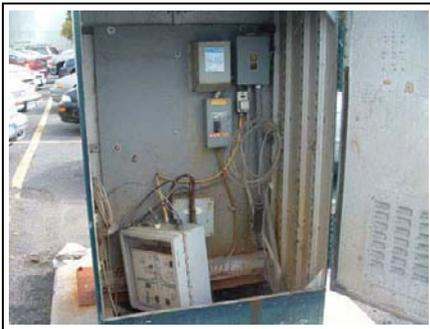
**Photo 9:** Well and control panel for former Hess Tank 2108 recovery system
