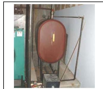
**Photo 12:** Fuel Oil Tank and Secondary Containment in Fire Suppression Room.
