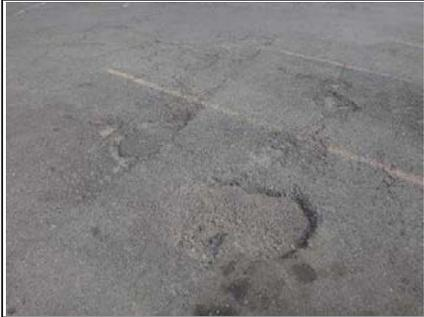
8. Potholes and deteriorating parking area asphalt paving.
