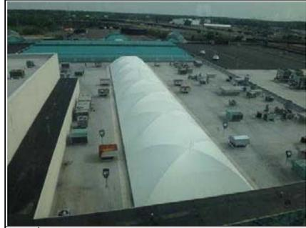
18. Teflon-coated fiberglass fabric roof area.
