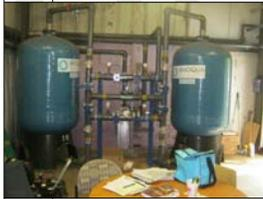
21. Filter tanks for groundwater treatment facility.
