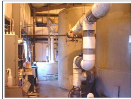
**Photo 4:** Interior of water treatment building showing process tanks and piping.
