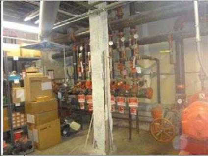
39. Sprinkler system control valves and electric fire pump.
