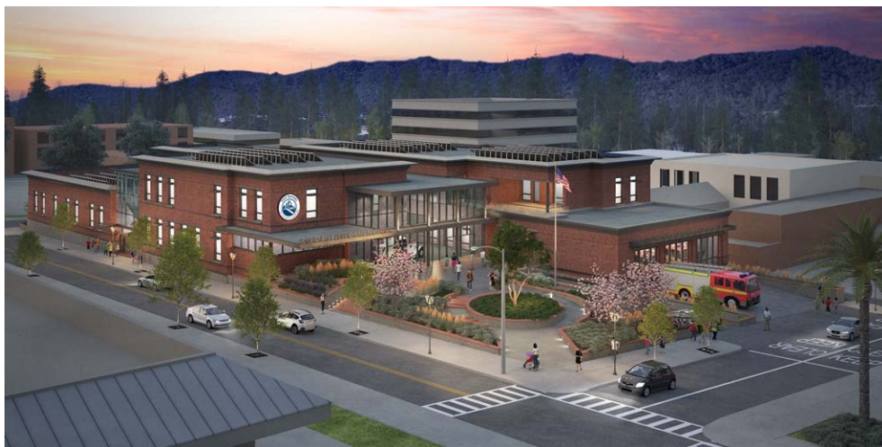
Public Safety Center
