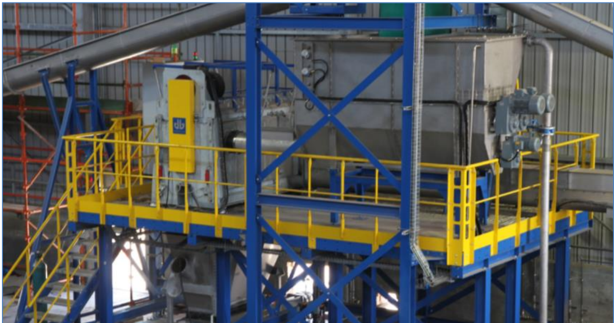
Figure 2-10 Anaergia’s Dynamic Cyclone for Organics Polishing
