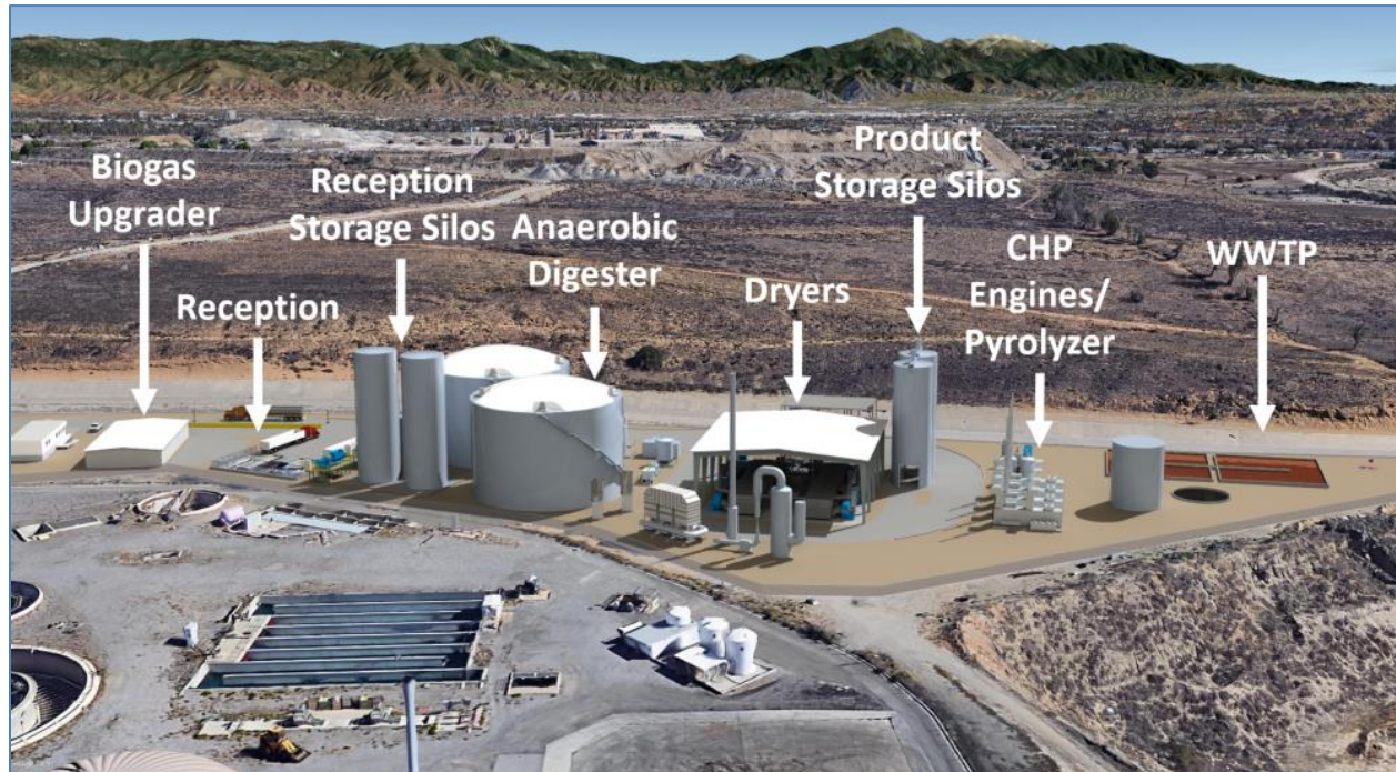
Figure 2-13 Proposed RBF Site at Full Build Out
