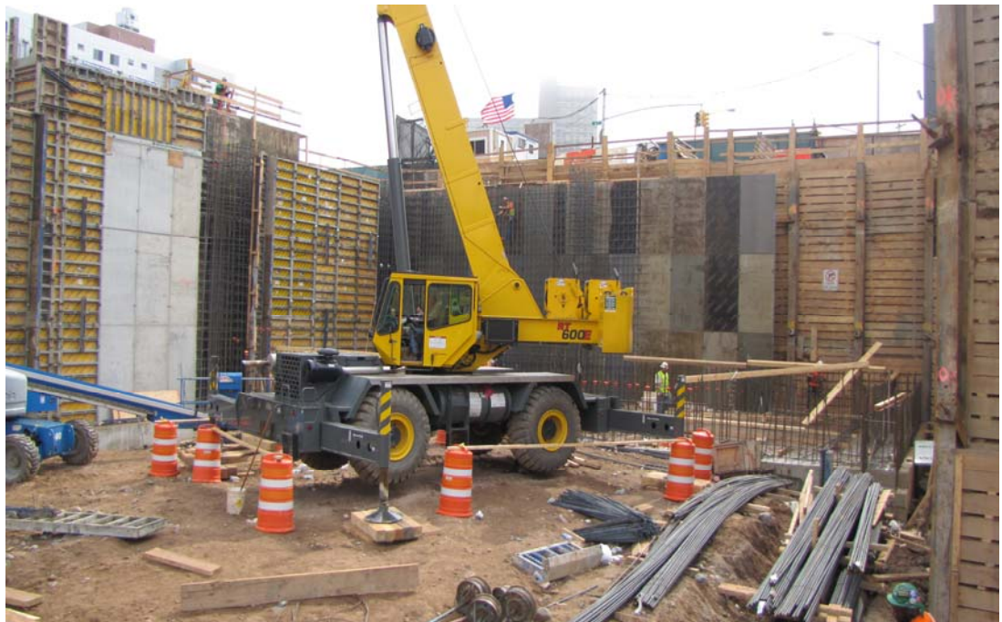
4. Formwork and reinforcing for foundation walls on Dean Street
