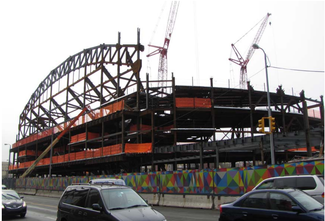
10. Roof truss section and structural framing along Atlantic Avenue
