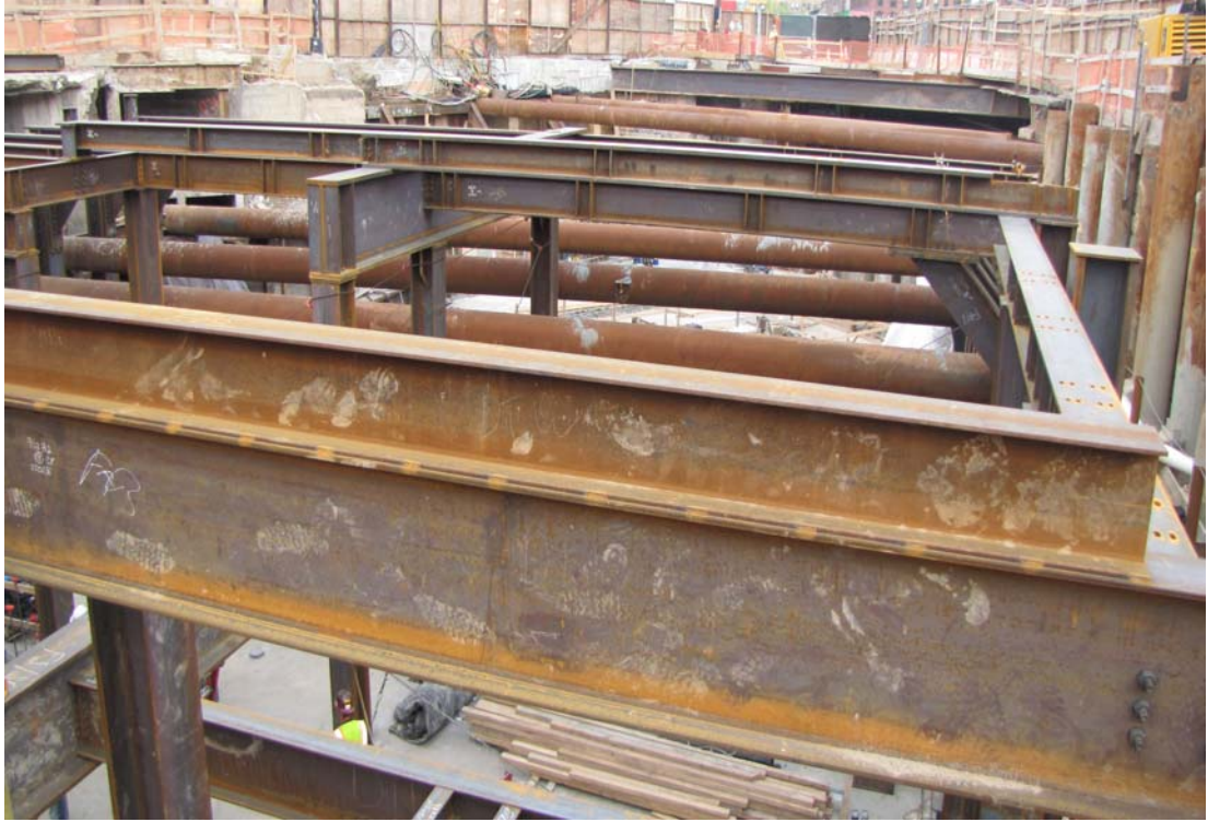
1. Steel framing at grade level for transit connection
