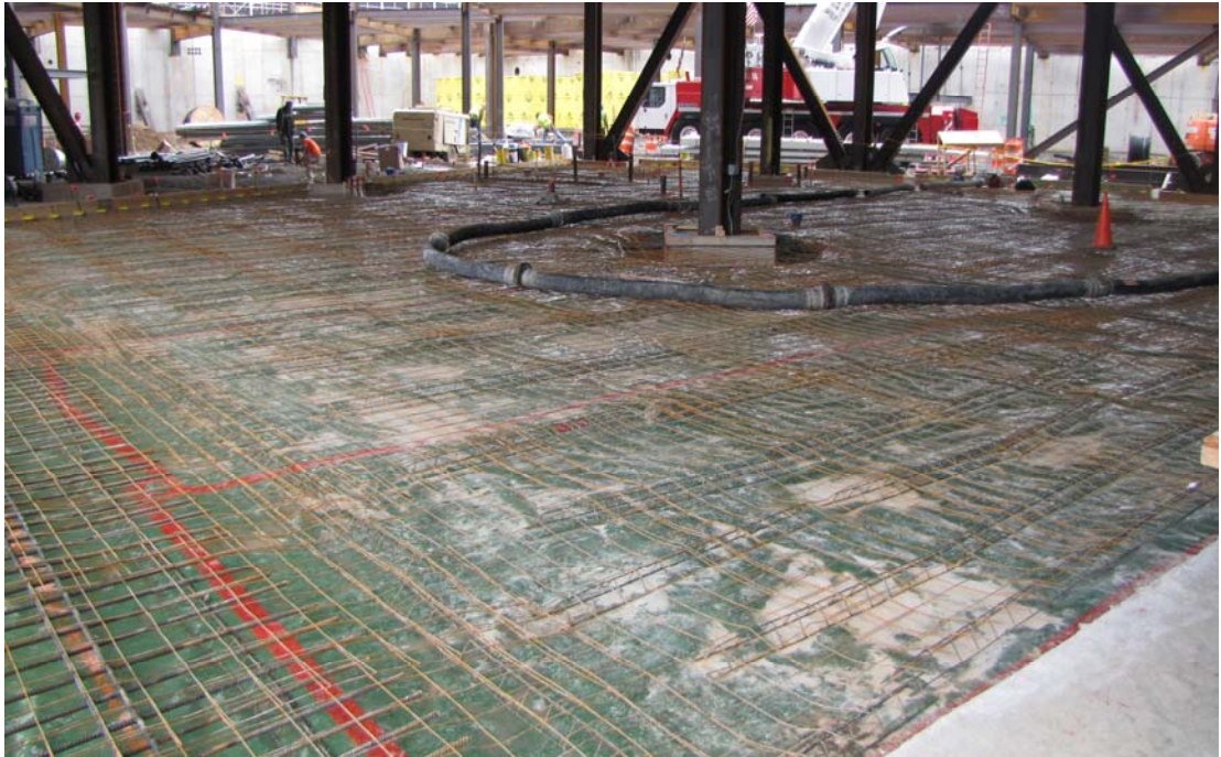
7. Reinforcing and wire mesh at slab-on-grade
