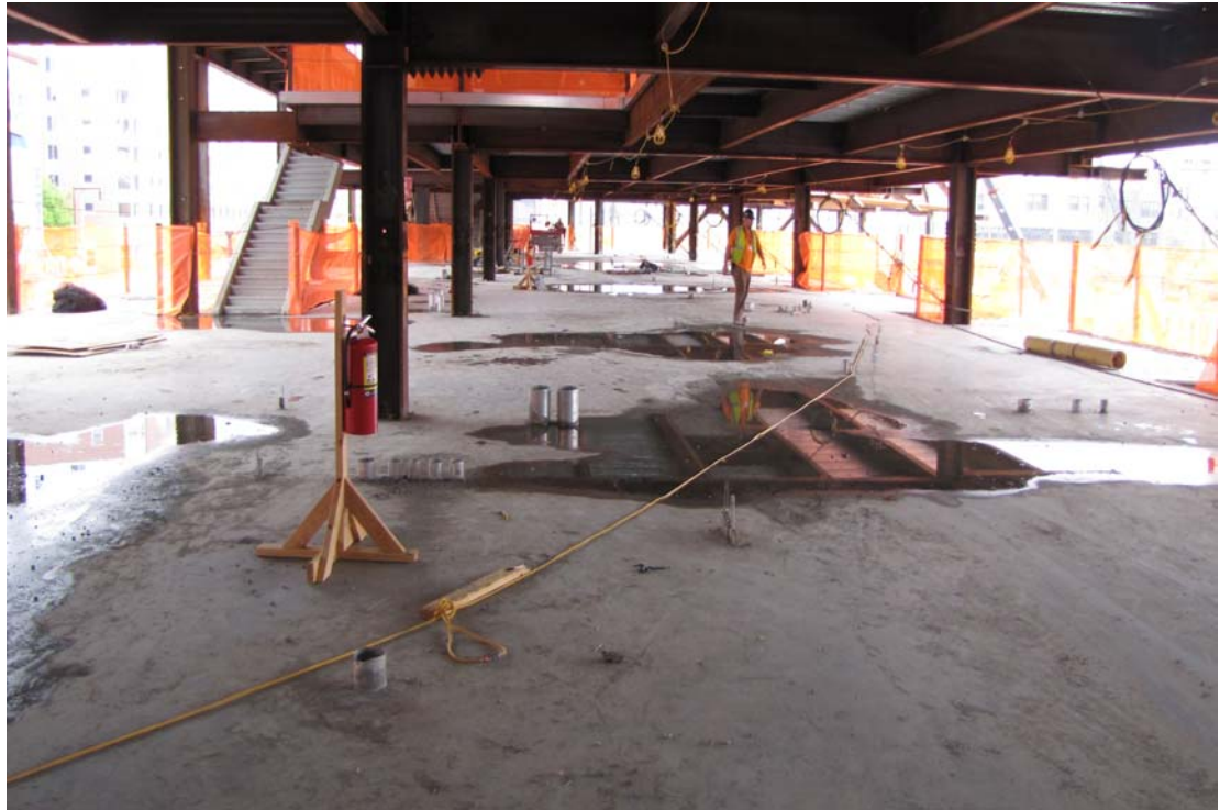
9. Slab-on-metal- and -deck at concourse level
