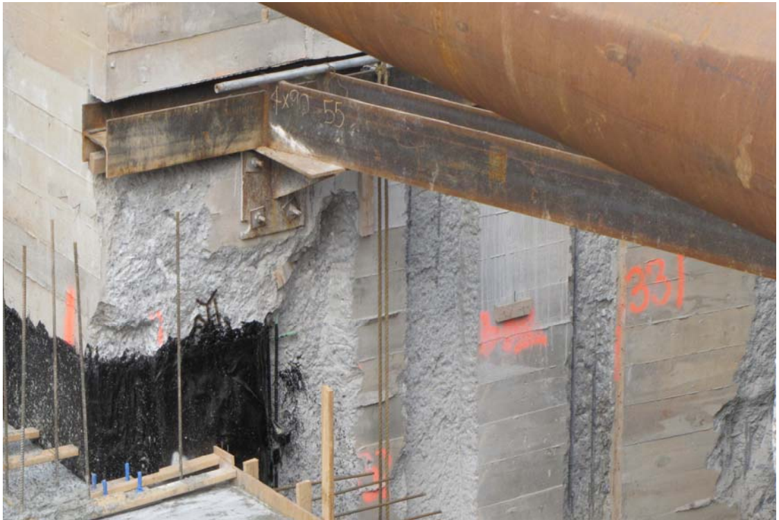
2. Underpinning along IRT subway wall
