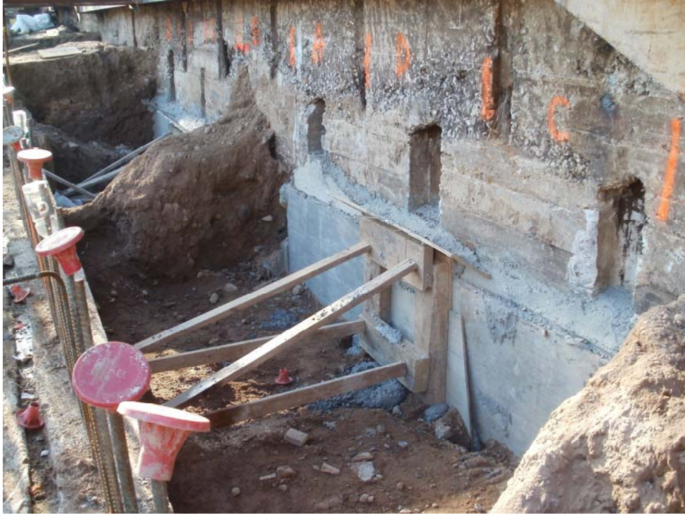
3. Underpinning at existing wall abutting MTA structure
