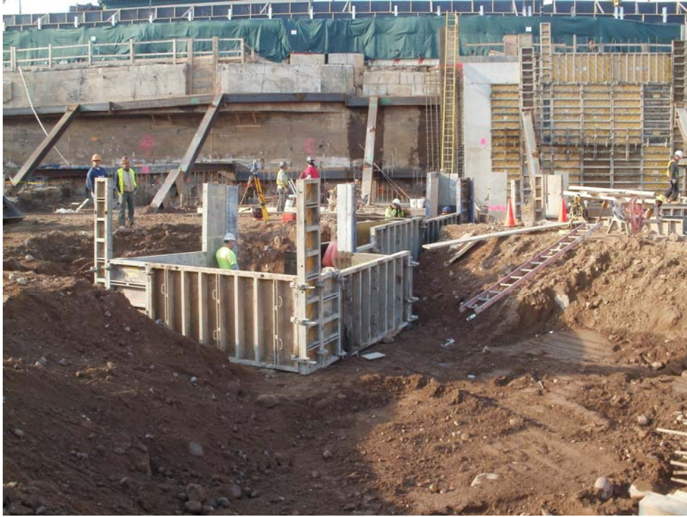
1. Formwork for interior footing at Line 1
