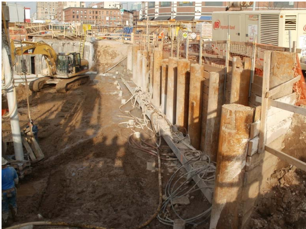
8. Piles driven along Atlantic Avenue at transit connection site
