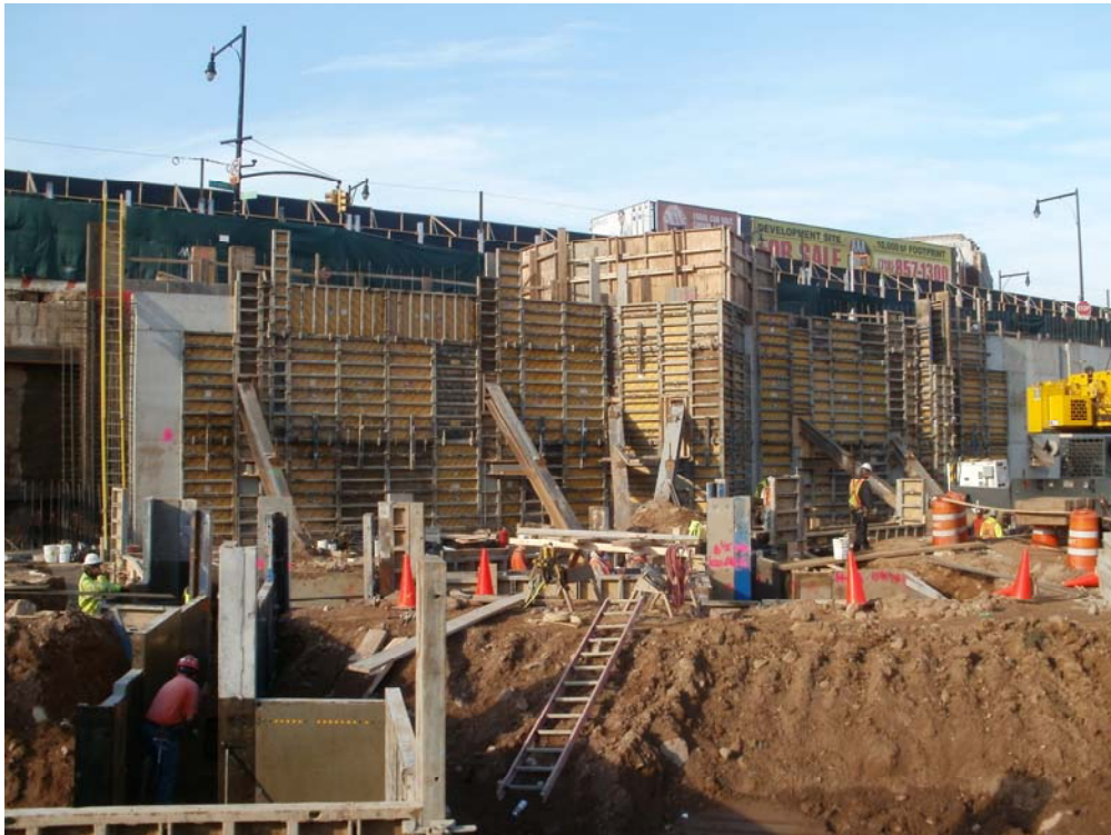
2. Formwork for foundation wall along Flatbush Avenue
