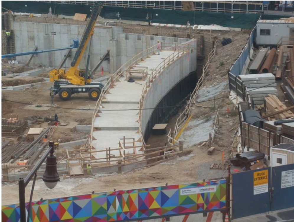
5. West retention tank concrete
