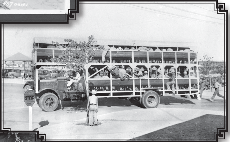
"Jumbo Rigs," like the one shown here, were used to facilitate faster drilling for the tunnels of the Boulder Dam. They consisted of scaffolding mounted onto a truck bed that allowed drillers to work on three levels simultaneously.
