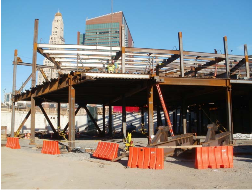
7. Structural steel started on lower suite level
