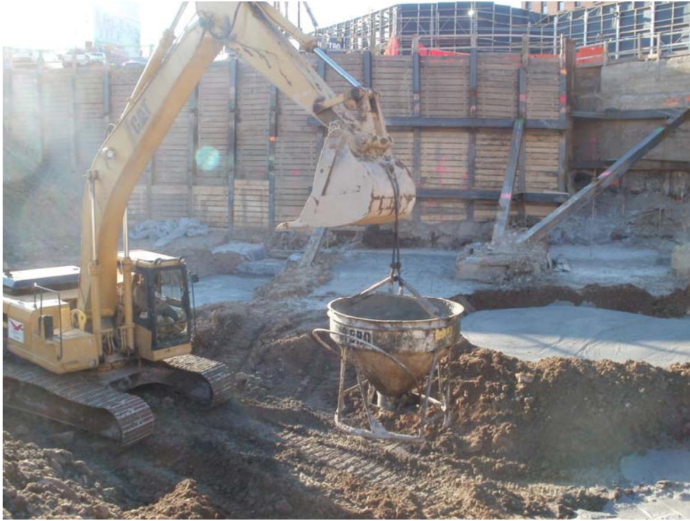
3. Mud foundation at southwest corner of site
