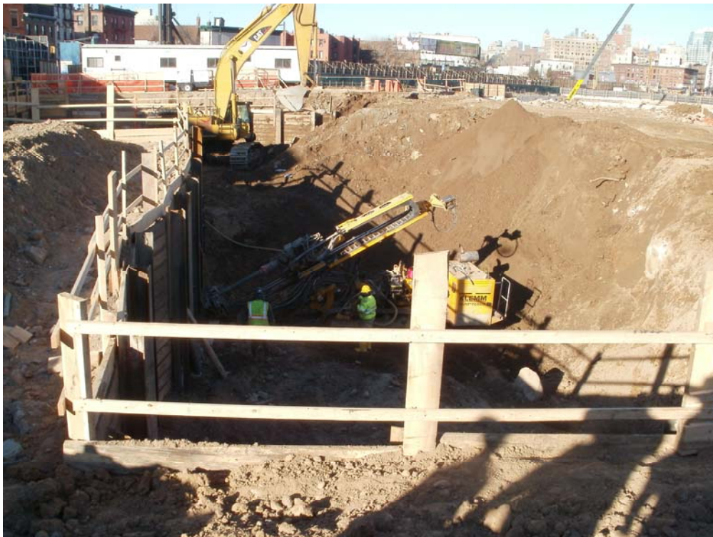
4. Tie-back drilling on Dean Street along south wall
