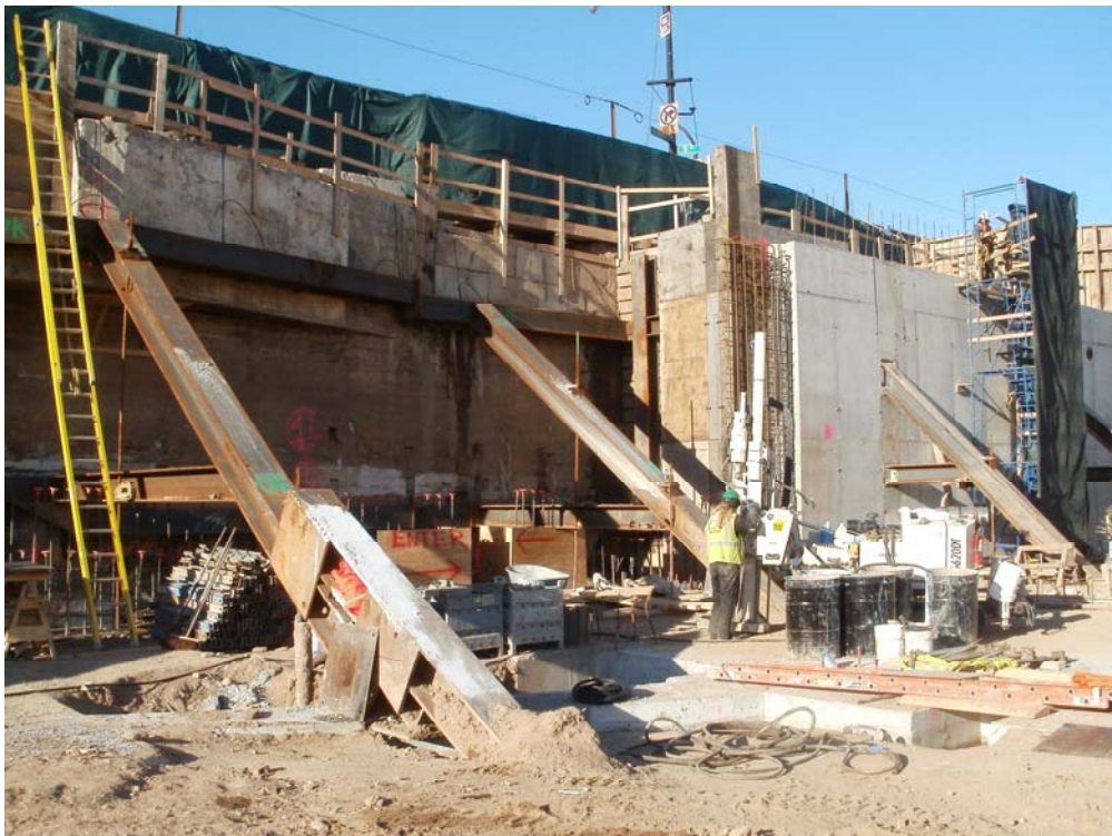
6. Steel beam braces with walers supporting the wall along Flatbush Avenue
