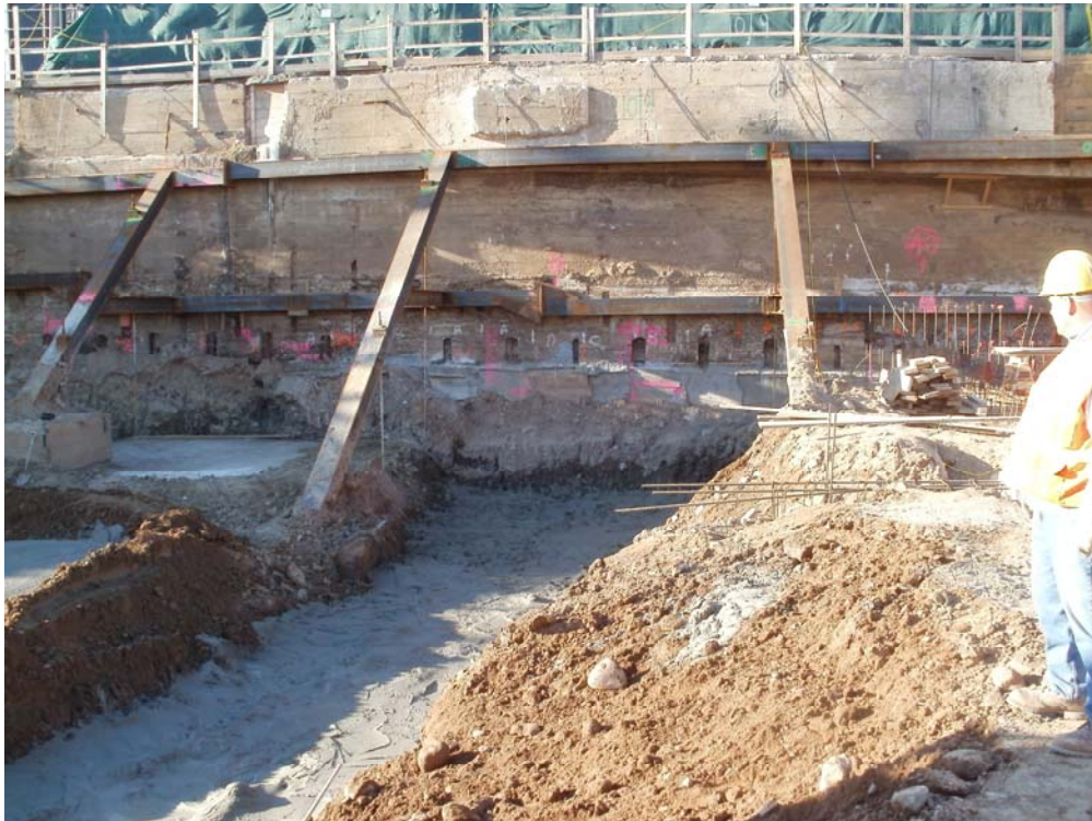
8. Underpinning at existing MTA foundation wall on Flatbush Avenue
