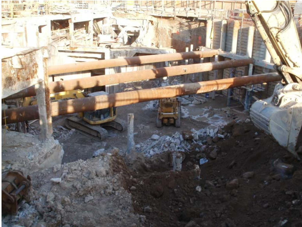
1. Cross bracing at excavated area of the transit connection
