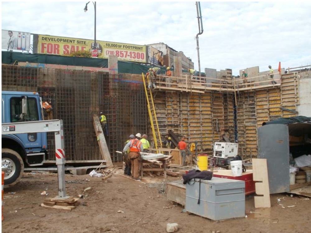
4. Formwork and reinforcing at foundation wall along Flatbush Avenue
