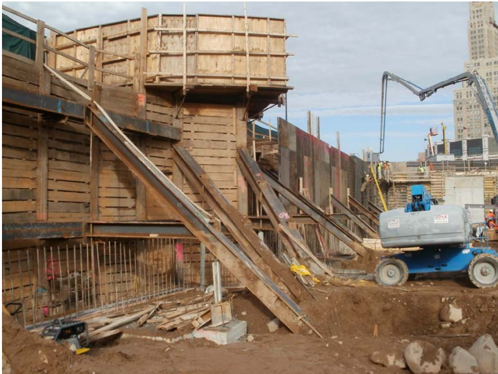
2. Walers and steel bracing along Flatbush Avenue
