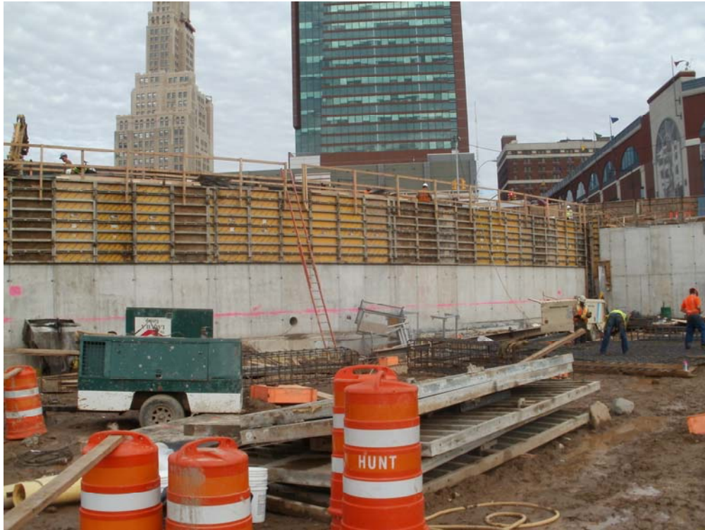
3. Retention tank concrete wall
