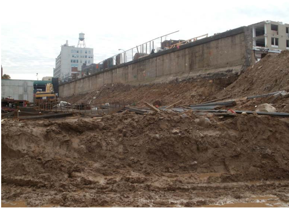
5. Soil berm along retaining wall
