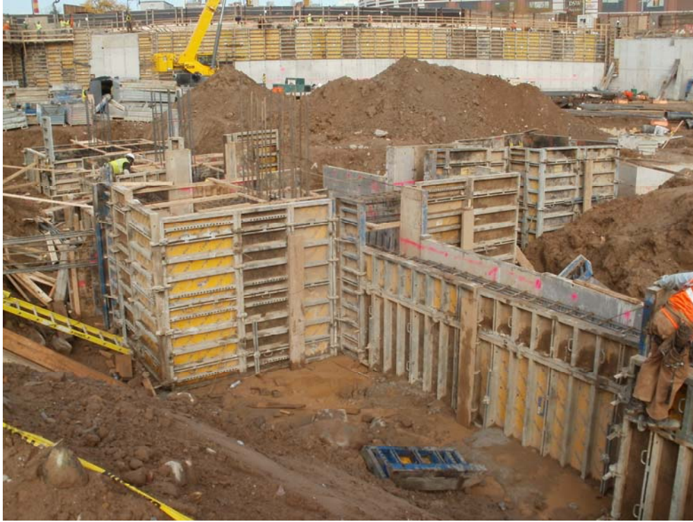
1. Interior footing formwork and reinforcing
